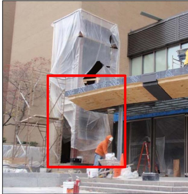
**Figure 5** Opening Created for Micropile Drill Rig
