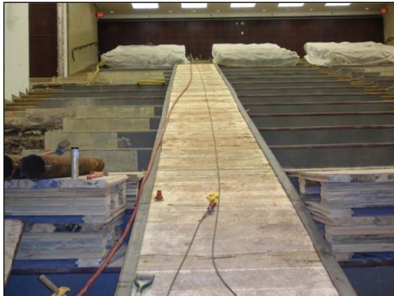
**Figure 6** Track/Ramp used for Micropile Drill Rig
