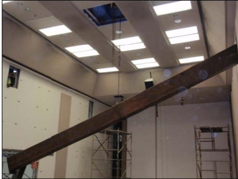
**Figure 8** Steel Column Being Lifted Through Existing Auditorium Roof
